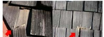
Areas of transition of upper and lower roof(s) and fascia need flashing and or repair.
