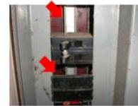
**Openings noted in the dead front cover. This is a safety hazard.** Correction is needed. Breaker handle ties appear to be home made We recommend a licensed electrician make further evaluation and corrections as needed before the close of escrow on the home.
