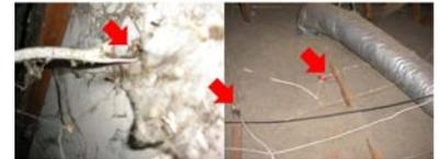
**WIRING NOTES:** Conductor(s) noted in various area(s) that should be reinstalled properly = safety hazard.
